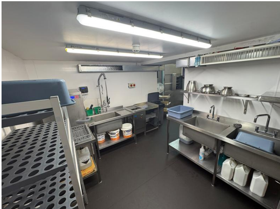
First Floor Side Kitchen Area
